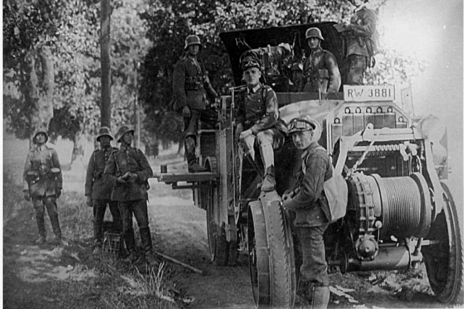
A motorized gun platform weighed 11.25 tons. Each vehicle had a crew of nine men. Each motorized gun battery comprised four Sd. Kfz. 1s. (CK)
