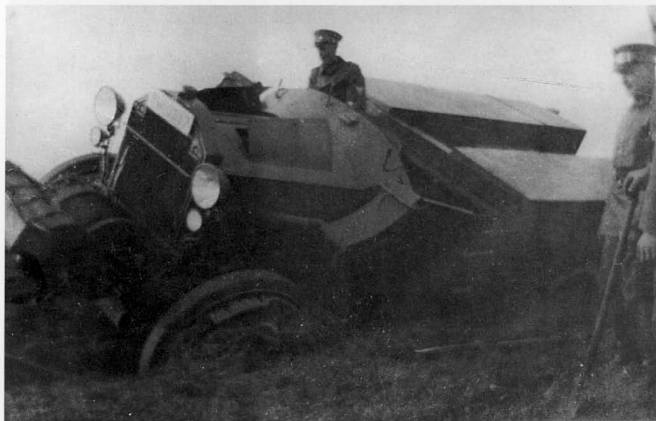
Above and below: The motorized gun batteries also found use for the KD-1 prime movers as ammunition transporters and recovery vehicles.
