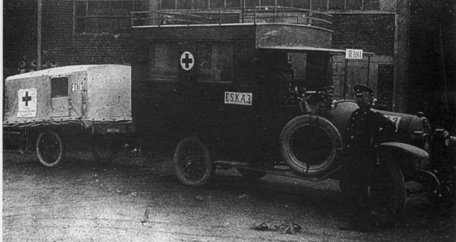
A Dürkopp ambulance with trailer, photographed after factory acceptance. Despite the existing fuel and rubber shortages, vehicles of this type remained in use with the army medical services throughout the First World War. (WF)
