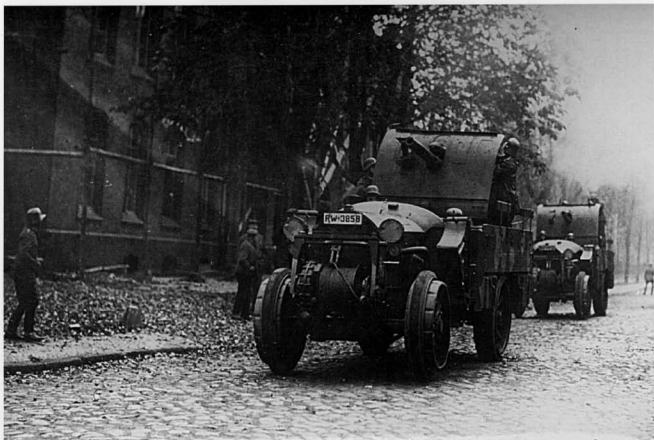
A motorized gun platform weighed 11.25 tons. Each vehicle had a crew of nine men. Each motorized gun battery comprised four Sd. Kfz. 1s. (CK)
