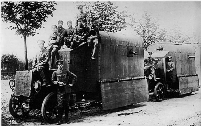
Two armored cars of improvised construction based on cargo transport chassis, being used by Freikorps troops. The combat value of such vehicles, which as a rule were fitted with untempered steel sheeting, remained low. Their existence stimulated the Reichswehr into creating armored wheeled vehicles; just as critical, though, was the analysis of operational experience. (WF)
