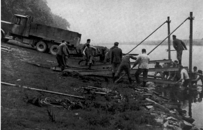
A Büssing-NAG Typ 3 GL 6 6x4 3-ton medium all-terrain cargo truck with an Sd. Ah. 14 attached. Engineers are standing by, waiting to offload the bridging equipment and assemble the bridge approach. (WF)
